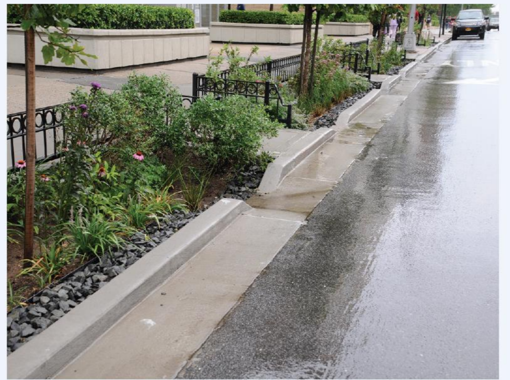
Curbside bioswales, NEW YORK, NY
